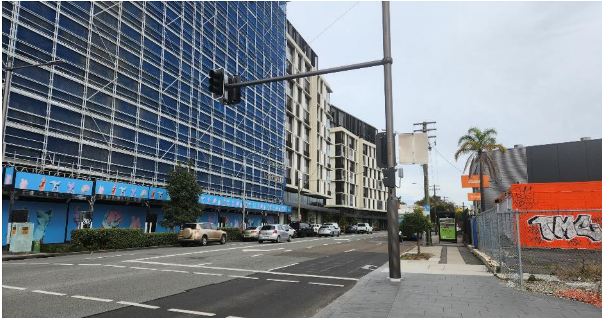
Figure 10: View looking south along Botany Road
